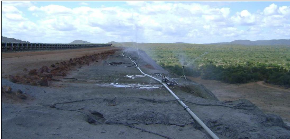
**Figure 19: Dust suppression system at Matimba Power Station**
