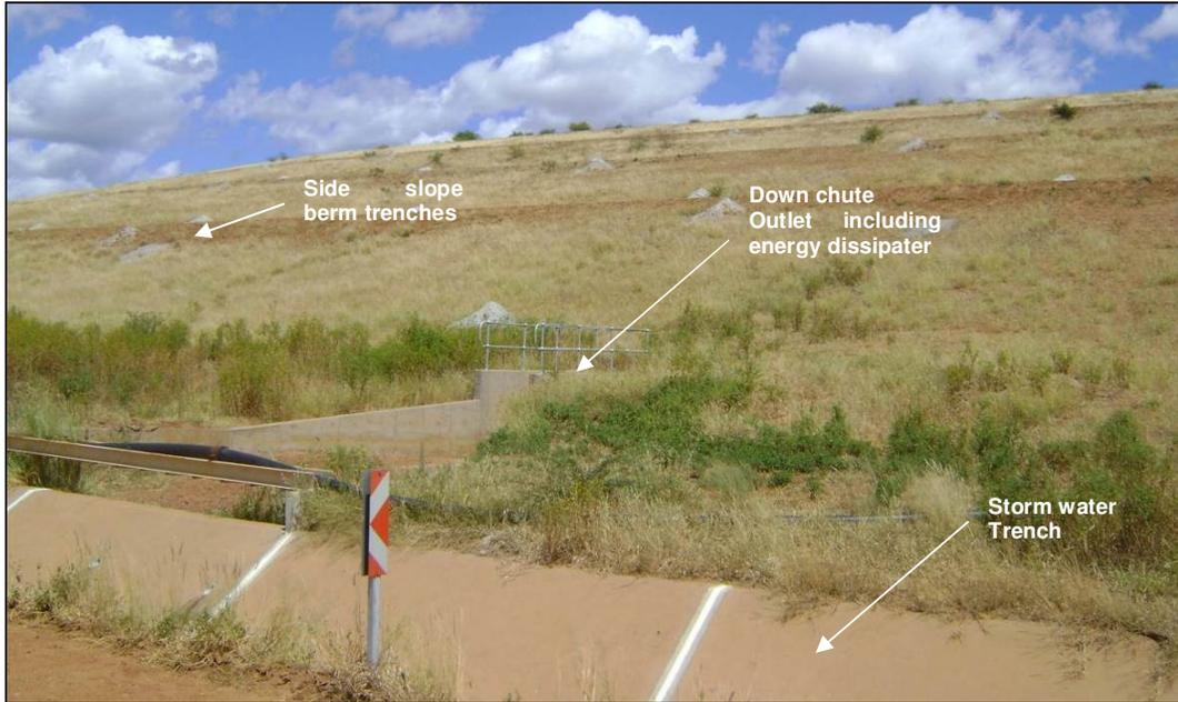
Figure 10: Rehabilitated area on Matimba Powerstation Ash Facility
