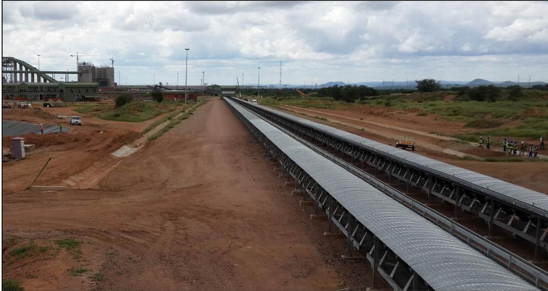
**Figure 7: Overland Conveyor Platform and storm water management infrastructure**
